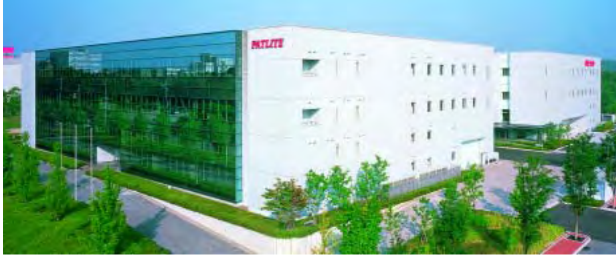
Manufacturing Plant, Japan
