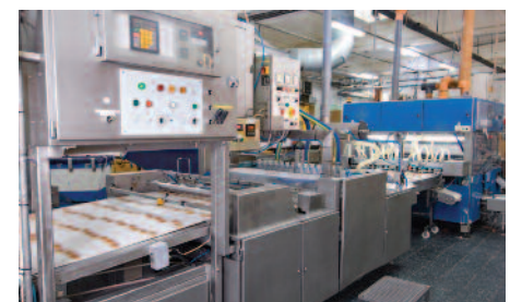
Plant floor data networks
