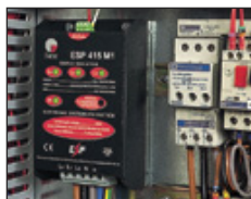
ESP 415 M1 installed within a control panel on the mains input to protect the panel's control systems. Note the remote indication connection (top of protector)
