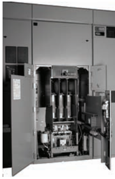
50L7 Vacuum Retrofit
