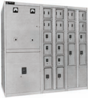
WRI Switchboard with Individually Mounted Molded-Case Breakers
