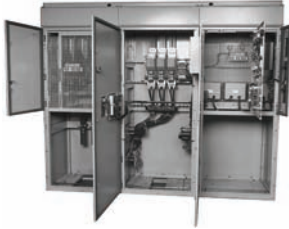
600V, NEMA Size 8, Synchronous Starter
