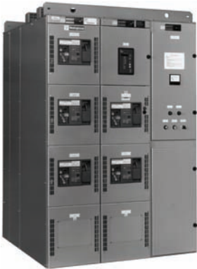
Pow-R-M-S/F Switchboard with Fixed SPB Breakers
