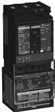
I-Line ™ J-Frame with ELM installed
