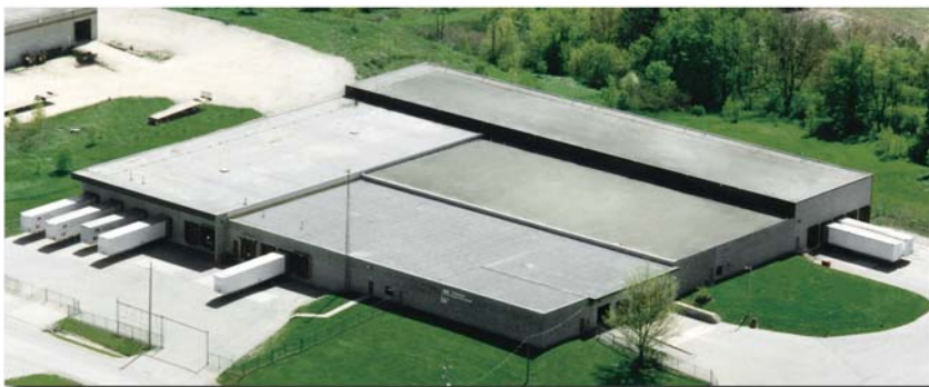
Hammond North American Distribution Centre
