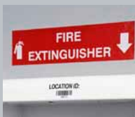
Safety Labels ...and many more!
