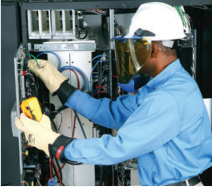
Proper preventive maintenance reduces the risk of UPS failure through thorough inspection, cleaning, testing and calibrating various electronic and mechanical components.
