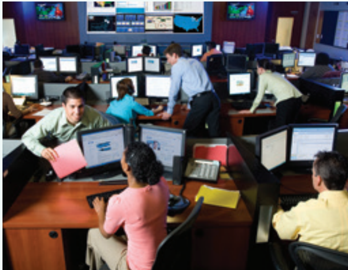
Eaton's Remote Monitoring Command Center is available 24x7 to monitor the health of your UPS.
