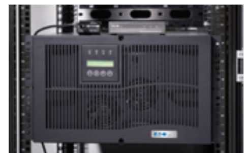
Environmental Monitoring Probe and Environmental Rack Monitor mounted on top of Eaton UPS
