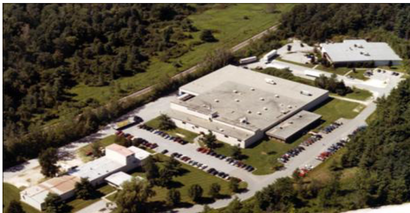
Harbour Industries Facility in Shelburne, Vermont.
