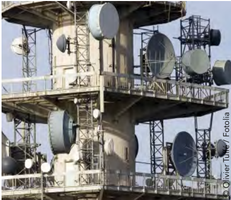
Telecom - Data infrastructure
