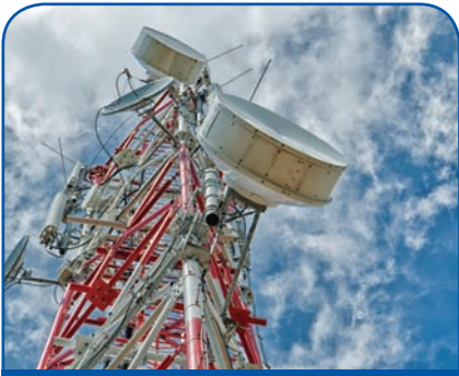
Telecom -Data Infrastructure
