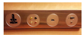
In-room multi-port electric outlets
