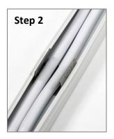
Secure with a masonry fixing, before feeding in the cables
