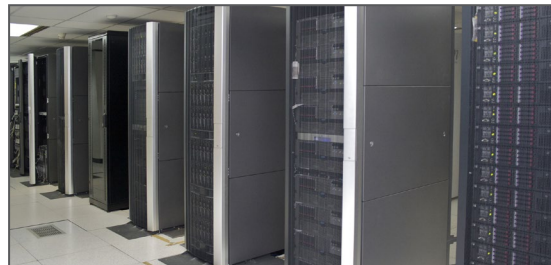
(Data Center Switches, Routers and Hubs)
