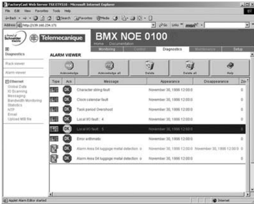
Alarm display from the diagnostic buffer
