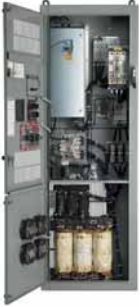
Enclosed 18-Pulse Drive
