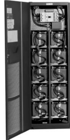
IBC-S with Door Opened—IBC-S is Compatible with Battery Types B12, B17 and E20
