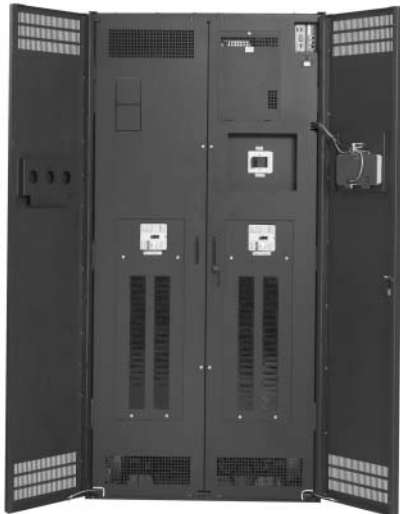
Power Distribution Unit
