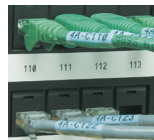
Patch Panel Labels
