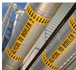
Pipe and Valve Marking
