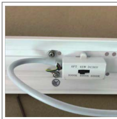
Internal CCT Switch
