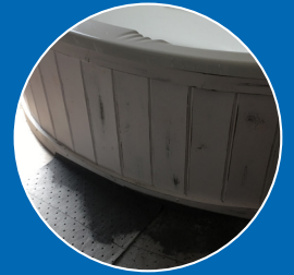
Leaking Pipe Work
