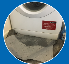
Leaking Washing Machine
