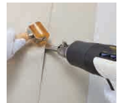
Welding PVC sheet Use of nozzle holder and spatula type nozzle along with roller
