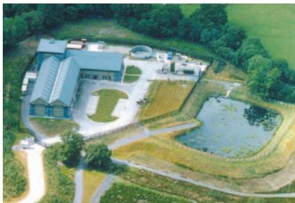
Example of remote pumping station.
