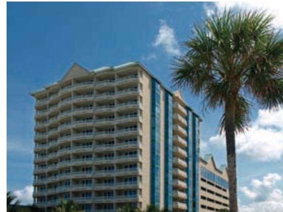
A total infrastructure solution was needed that could handle a load of approximately 60 kW.
