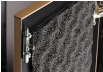
Acoustic foam lining reduces noise by 15 dB.
