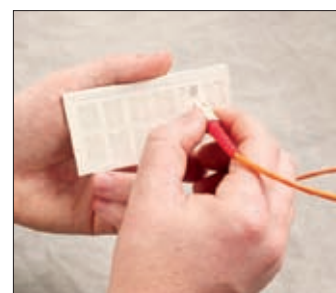
Solvent from a fiber optic solvent pen, applied to a special purpose, disposable cleaning pad, is a best-practice method for cleaning fiber optic cabling.
