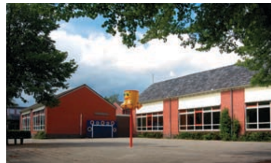
Schools need cost-effective, scalable cooling solutions to protect their IT equipment.
