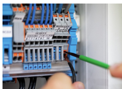
Conductor termination
