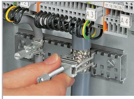
Securing an additional shield clamping saddle.
