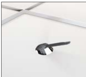
1. Insert the mounting support through the fixing hole.
