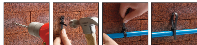
Fixing of Wall Plug Ties.
