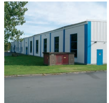
Warehouse- and production facility in Nässjö, Sweden
