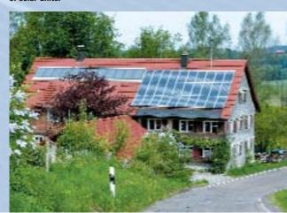
Connected since June 2006: The PV reference system, "Stoiadler III" with 200 modules and 26 KWp of power.
