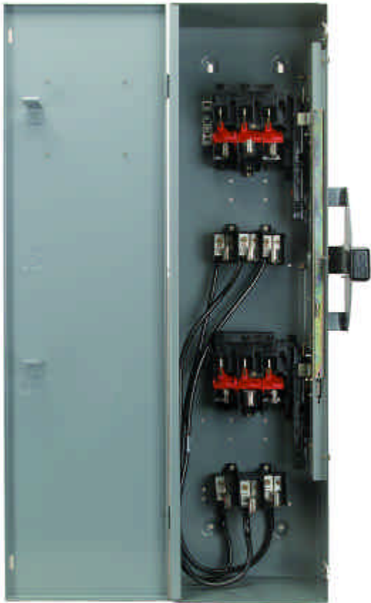
60A Fusible Double Throw Switch
