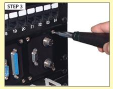
Using a Phillips or Flat screwdriver, install your sub-panels in the master rack panel.
