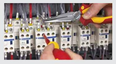
In addition the handle insulation and curved handle ends that prevent the fingers slipping away ensure even more safety.
