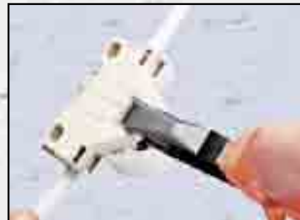
3. Close lid and squeeze with pliers till both "clips" latch.
