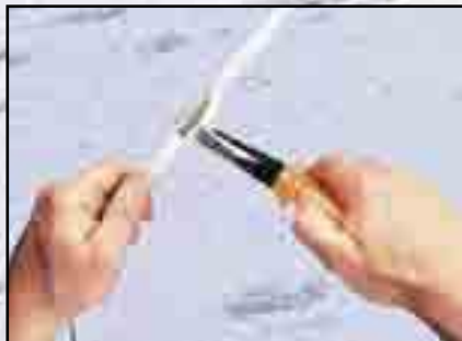
1. Remove outer sheathing only to required length.
