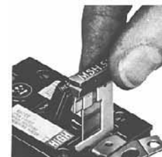
Heater Element Installation
