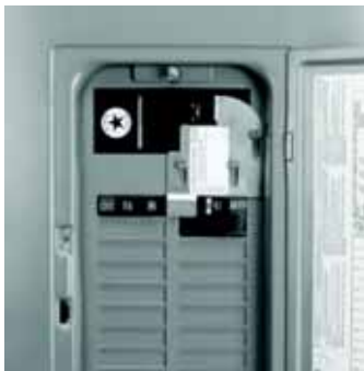
Cutaway Showing Installed Generator Interlock Kit
