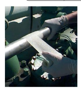
**Quick Wrap** has good temperature, pressure and chemical resistance and is quick and easy to use.
