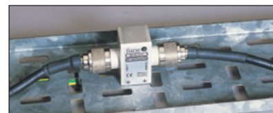
ESP RF 111121 on a coaxial cable running between an antenna and an RF receiver
