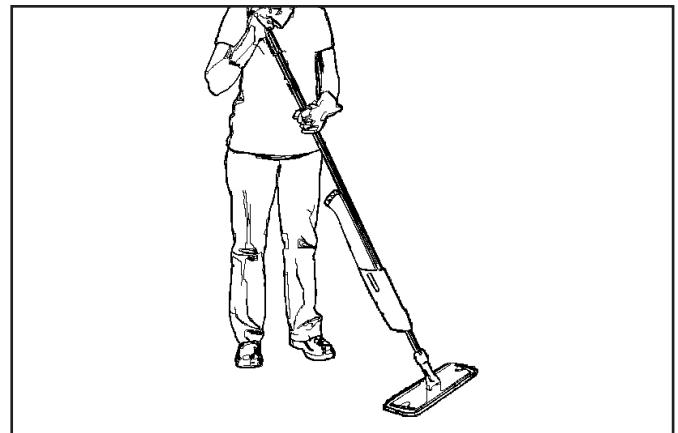
Figure 5. Applying floor finish with Flat Mop (optional).
