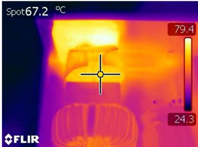
Figure 61 – Differential Mode Choke (L4), 115 VAC Input, 100% Load, Room Temperature.
