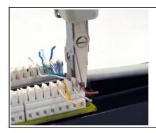
3) Using a suitable punch down tool, punch the wires down into position.
