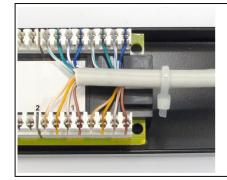
5) Repeat steps 1 to 4 for the required amount of cables and tidy them using cable ties.
