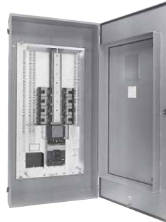
Access to Wiring Gutters
