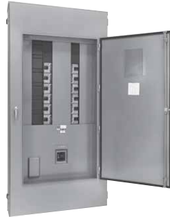
Access to Circuit Breaker Handles
