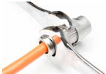
Step 17 - Tighten to 5-7 N/M using 25mm wrench
