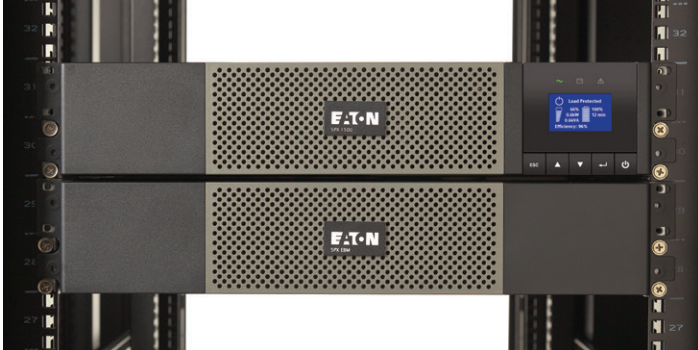
A UPS paired with an extended battery module helps extend runtime to meet service level agreements.
