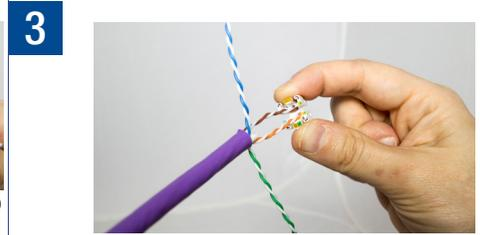
Locate the brown box on the bottom of the cable manager. Insert the brown pair and green (for T568A) or orange (for T568B) pair through the holes and begin sliding the manager down the cable
