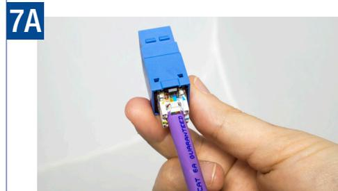
Align the rear jack latch with the latch on the cable manager and snap on your RJ45 housing. The terminated jack is now ready for testing.
