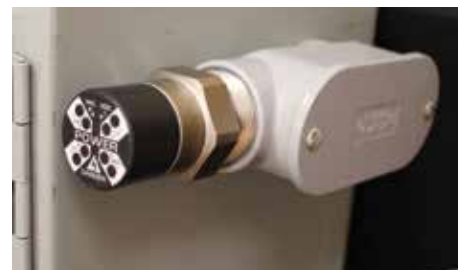
1 1/2 conduit vertical with R-3W
