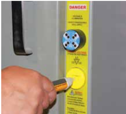
Fig. 9 Verifying proper operation of the NCVD
