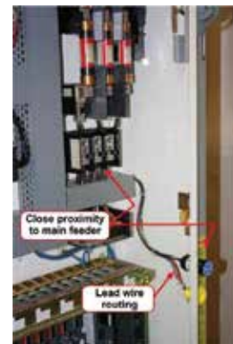
Fig. 6 Proper location of a three-phase portal
