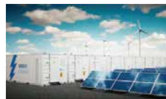
Energy Storage System
