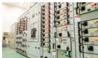
Power Distribution Control
