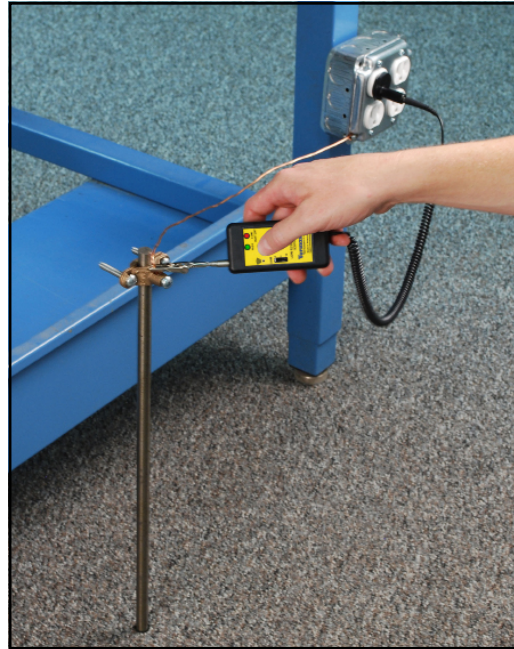
Figure 4. Testing auxiliary ground with the 222645 tester
