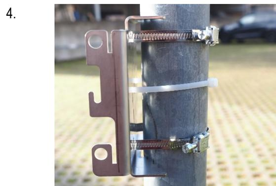
Once the mounting plate is installed, you can simply attach *Nuboo Monitor One* by sliding the system's backplate into the mounting plate. While the system is designed in such a way that the *Nuboo Monitor One* will stay in place from this moment, it is important to tighten the screws on the side to ensure safe and secure fixation of the system in all conditions.
