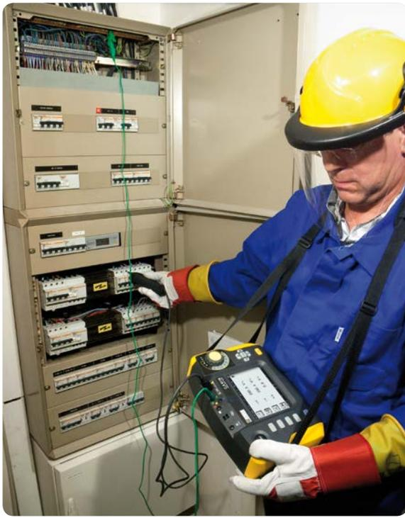
In domestic, tertiary or industrial environments, these new multi-function installation testers can be used to check an electrical installation's compliance with the applicable standards. This verification is mandatory to ensure that the installation is not hazardous, whatever the type of building tested (domestic, public building, industry, etc.).
