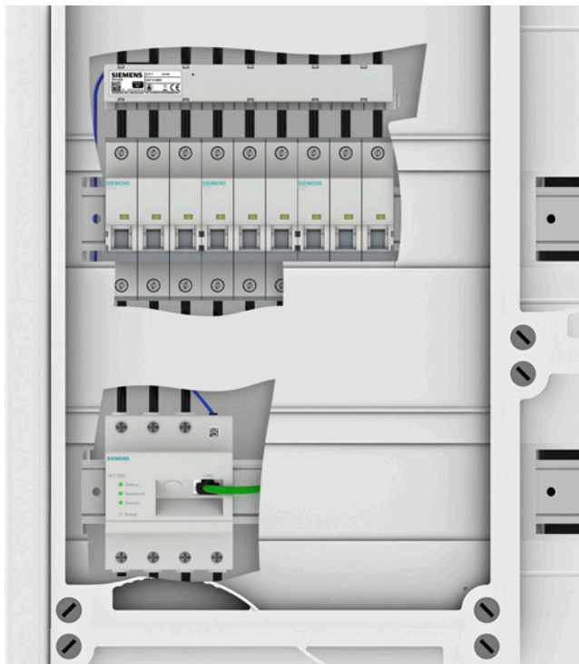
7KT PAC1200 multichannel current measuring system installed
